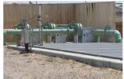
Contrast the corroded and exposed aeration basin at the more than 45-year-old wastewater treatment plant on Sara Road (top) with the clean enclosed one at the Cabezón purification plant (bottom).
