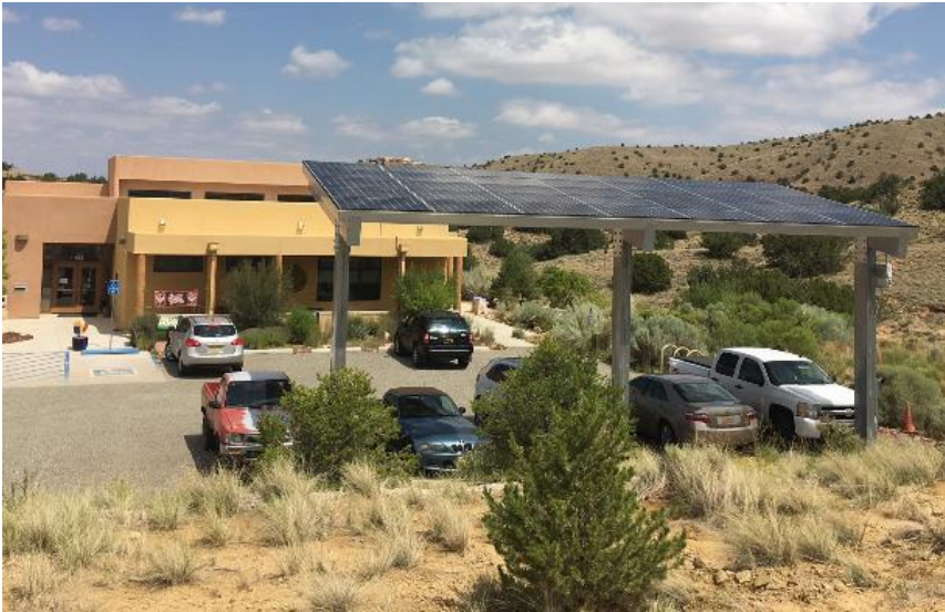
Placitas Library Carport Solar System
