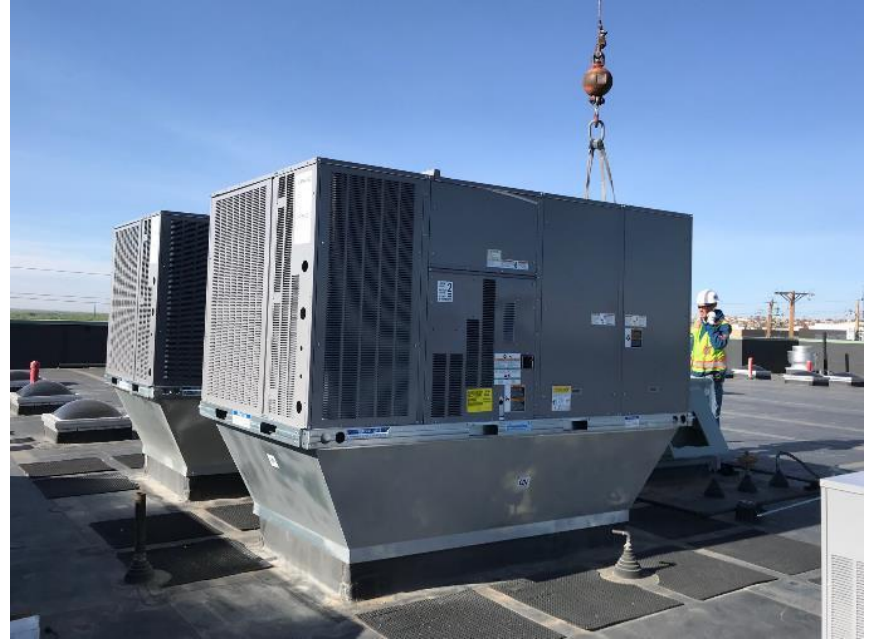
New RTUs- 6 & 7 Typical of 26 new units
