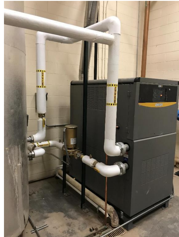
New Domestic Hot Water Boiler
