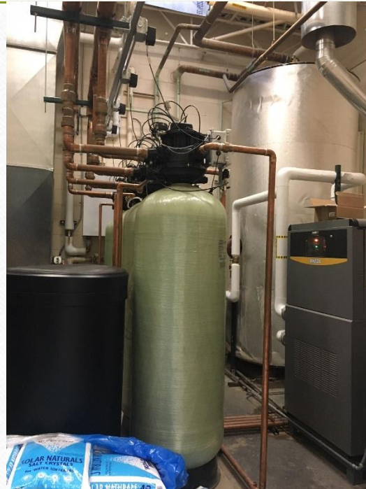
2 West Water Softener
