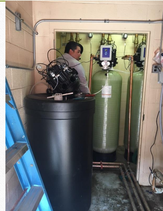
North Sally Port Water Softener
