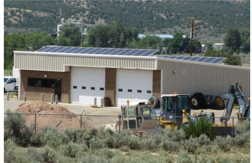
Cuba Roads Department Rooftop System
