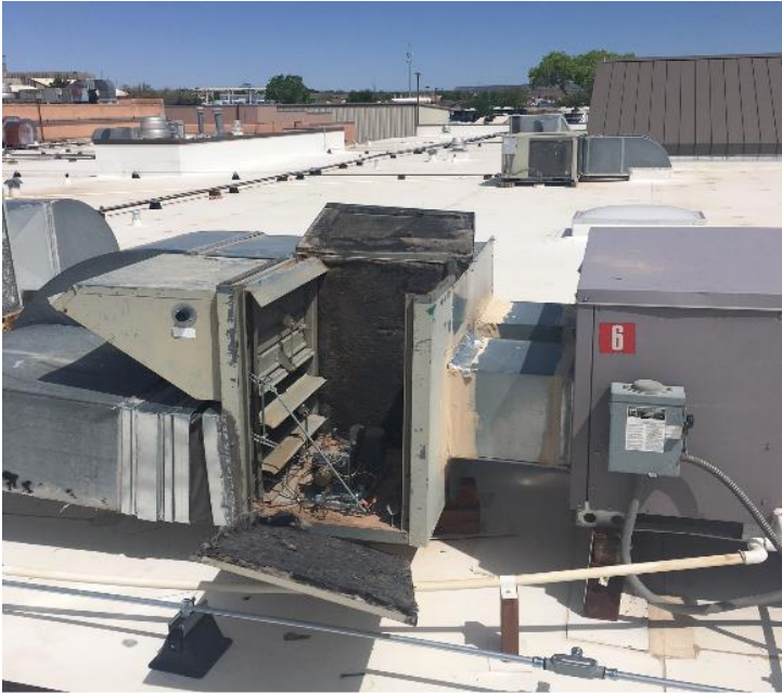
Old Rooftop HVAC Units
