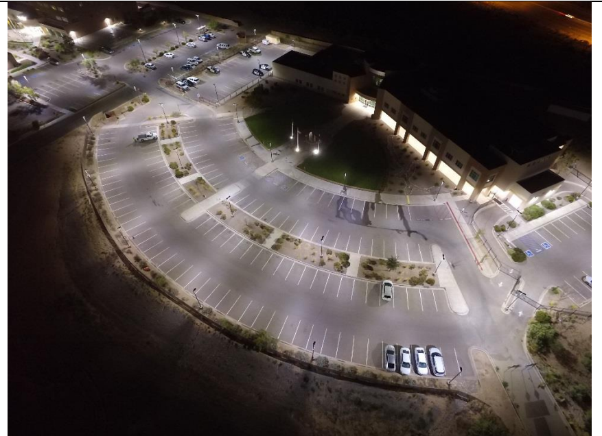
Judicial Court and Admin Parking areas with new LED lights
