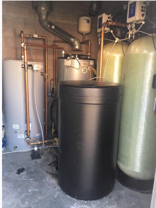
1 West Water Softener
