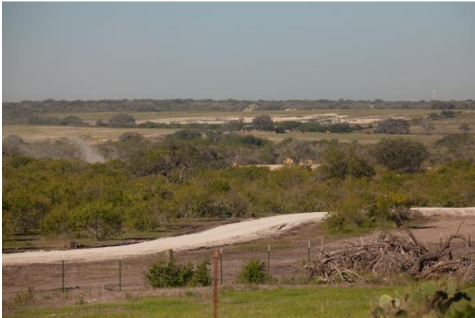
Clearing and grading take place for a new Marathon Oil fracking and well site in the Eagle Ford Shale, near Karnes City, Texas. (Lance Rosenfield/Prime)
