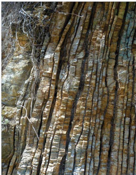
Figure 4. The highly fractured Monterey shale, exposed near the Hayward fault in Berkeley, California. Dark bands are black shale. Tectonic movements have brought this sedimentary rock to the surface and rotated the beds from horizontal to vertical. (Photograph by Eldridge Moores.)
